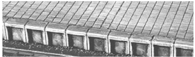
Low platform edge concrete and brickstone (above).
