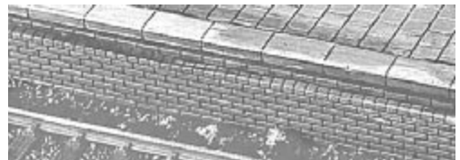
▲ High platform edge of brick. Surface of staggered 30 cm flags (Mould 2141).
