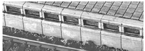
▶ High platform edge of concrete elements with step and top box.
