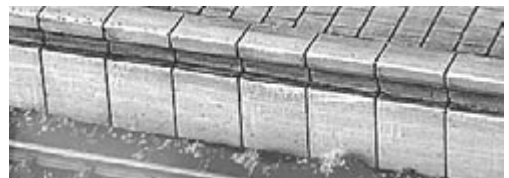
▶ High platform edge of concrete elements with step
