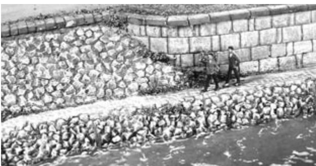
Left: Waterway embankment build with mouldset 6200 and stone rows from mould 6026
