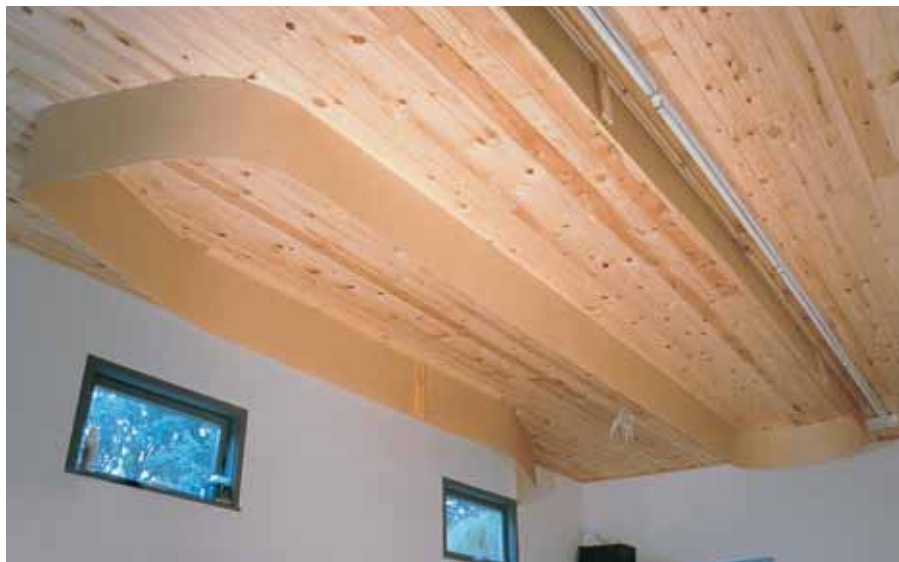
Fig. 1. Top of the frame. The valance, or the top part of the “picture frame,” is made from 1/8" Masonite and curves to match the projected contours of the layout.
