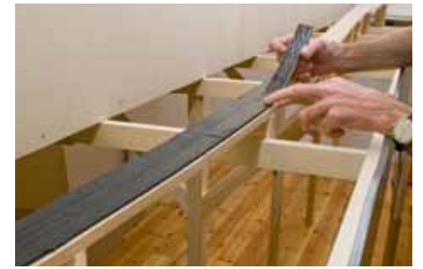
I applied the sound-deadening strips to the subroadbed. The asphalt-based sheets are self-adhesive, so you just remove the backing paper and apply it. Make sure that the surface you apply it to is free from dust.
