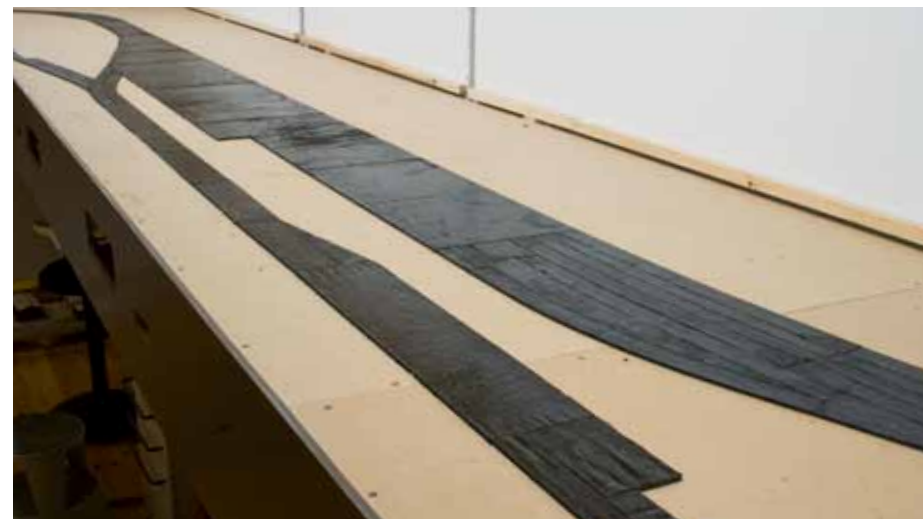
This picture shows the Daneville area with the sound-deadening material in place. On straight areas with multiple tracks, I used larger sheets instead of strips.
