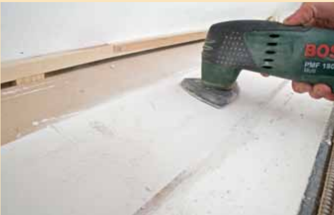
6. After several days, when the plaster had dried completely, I removed the foam tape and sanded the surface. A power sander is very effective. I learned that you have to move the sander constantly and never sand the same area for more than a few seconds or else you risk sanding away all of the plaster.
