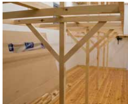
A view under the freestanding section. Having center posts instead of legs on each side of the frame makes the aisles feel wider.
