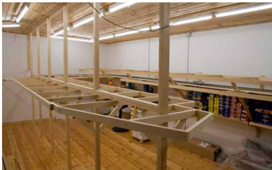
A view across the room with the freestanding section in the foreground and the Daneville area with the staging below in the background. I used 1 x 2s for the frame construction and 2 x 2s for the center posts in the freestanding section.
