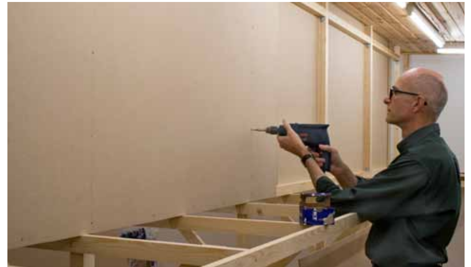
I mounted 1/4" medium density fiberboard (MDF) back to back on the posts as a scene divider and as a base for the backdrop.
